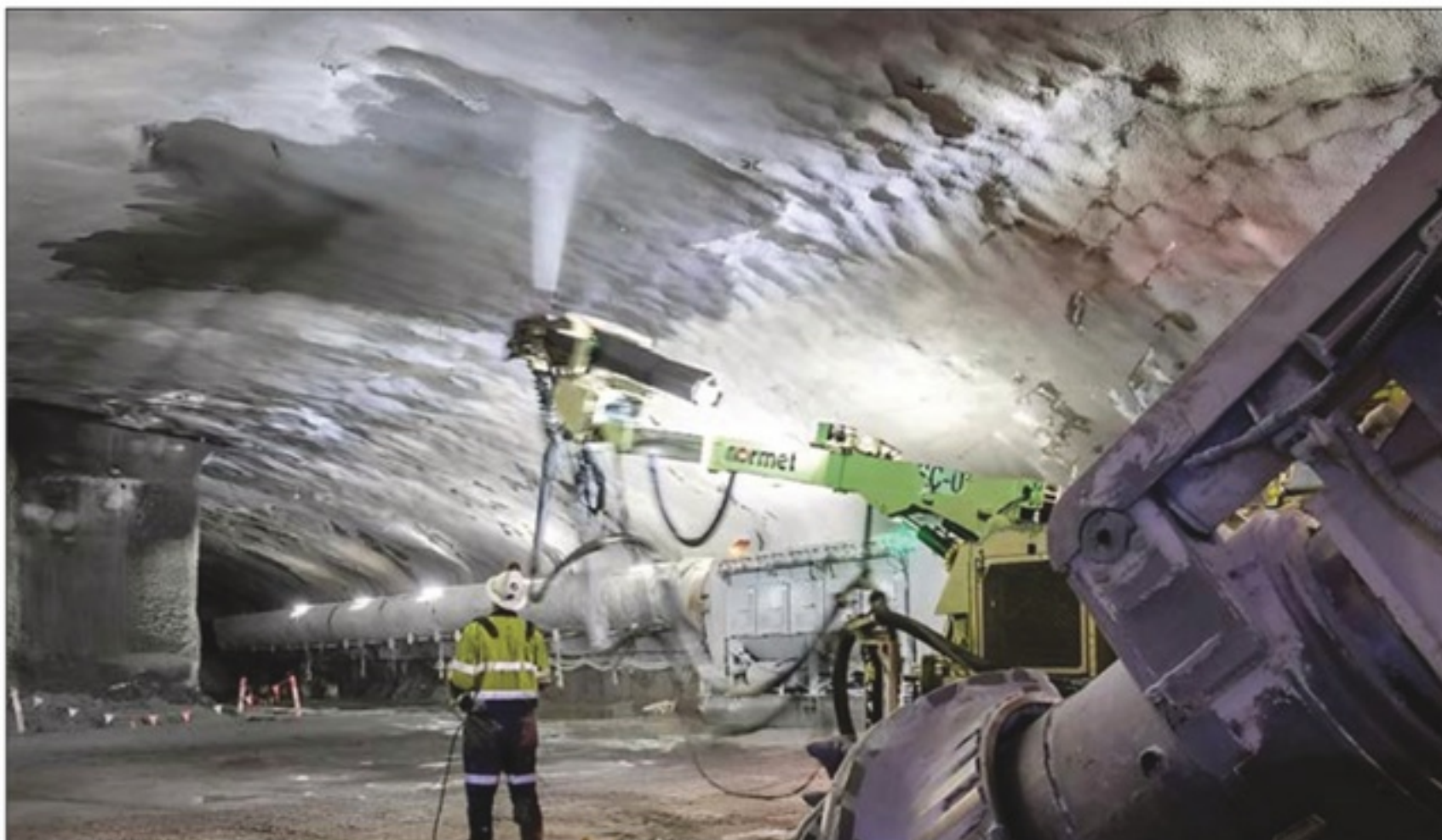
©West Connex M4-M5 Link Tunnels
